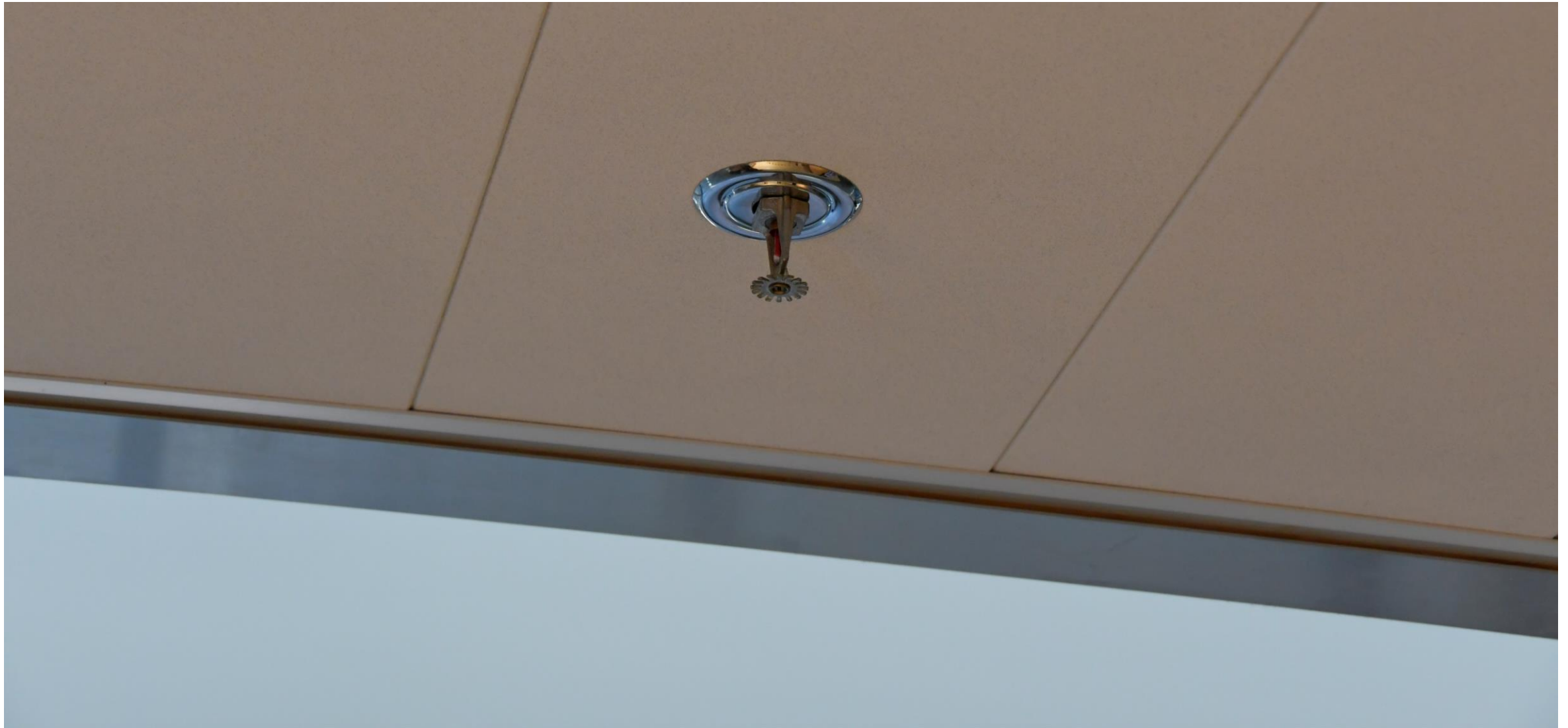
DSC0953 | sprinklerkop
